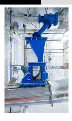
The Master BulkSlide is a solids flow meter that measures with accuracy from  $\pm$  0,5 percent. It can be used for most solid bulk products that are free-flowing and non-sticky. The BulkSlide calculates the product flow and total by measuring the force of the bulk product as it contacts the curved plate within the BulkSlide assembly.
